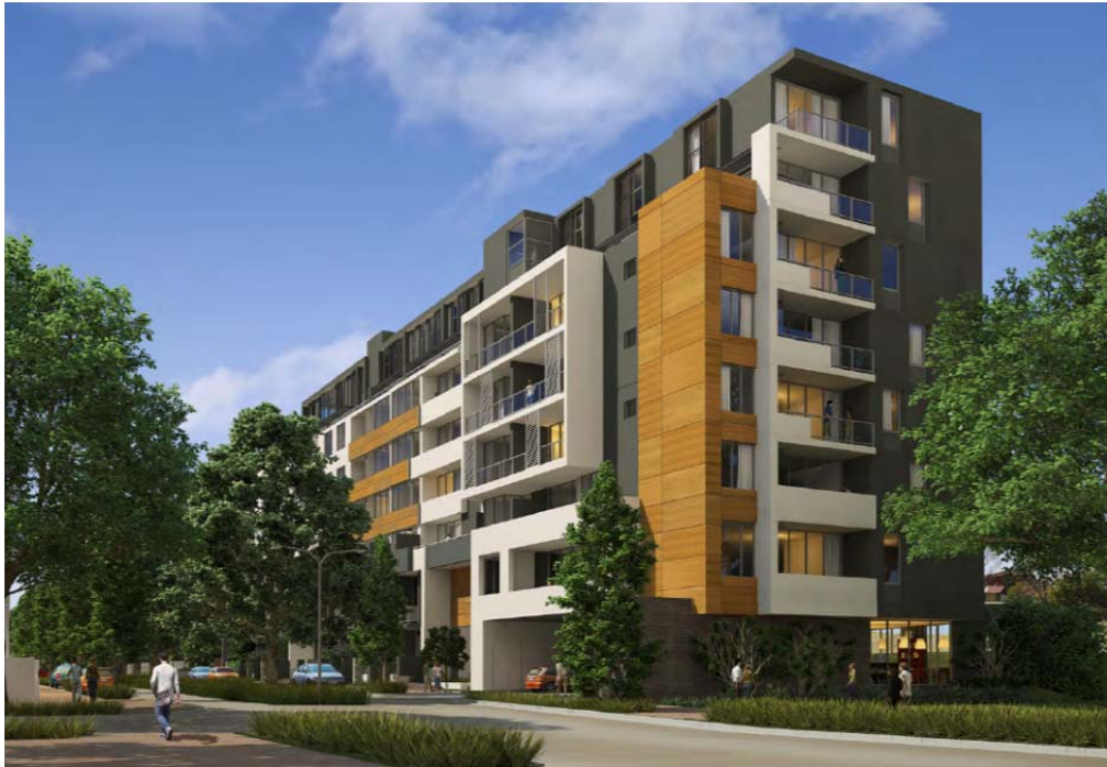
Figure 13 – Amended south-west corner.
