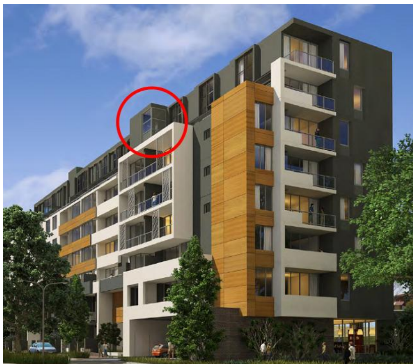
Figure 27 – External element to garbage room facing west (street).
