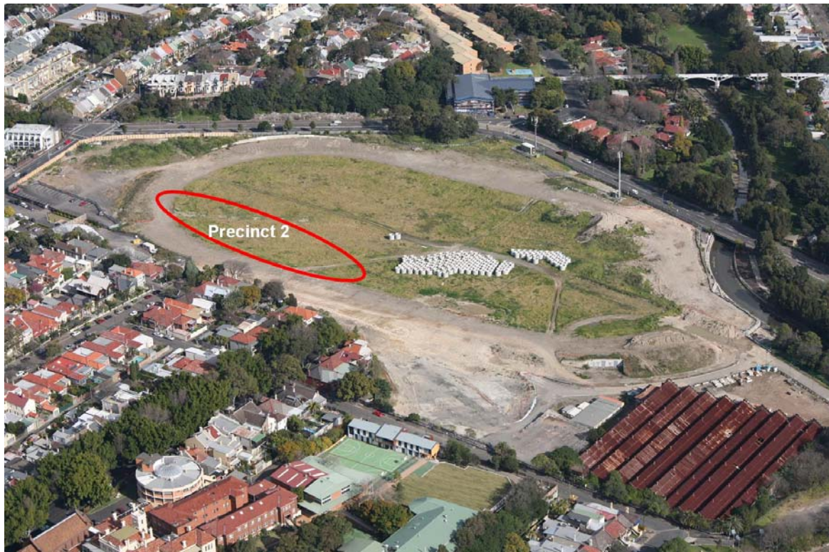
Figure 2 - Harold Park (looking west). The general location of Precinct 2 is shown circled. As shown in the aerial, the paceway, grandstand and other ancillary buildings have been demolished.
